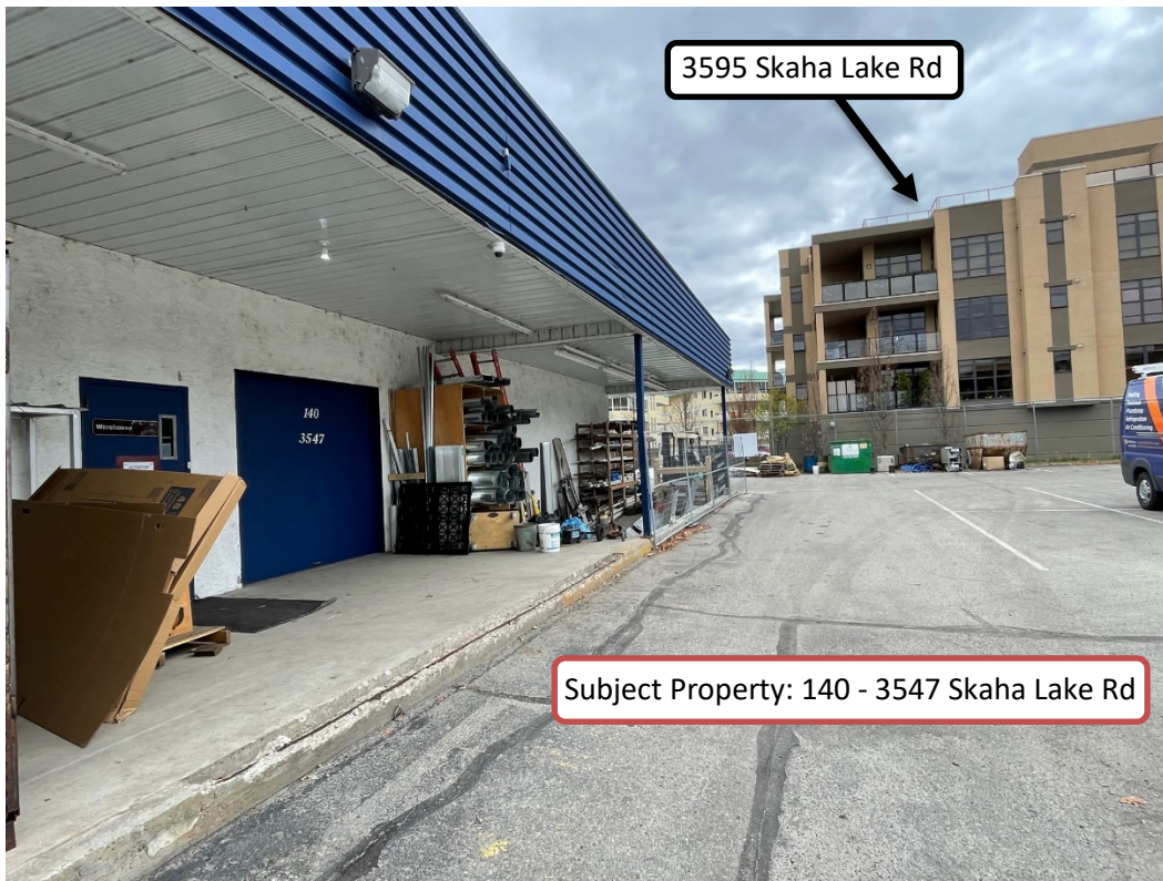
Looking south at the business from the subject property parking lot
