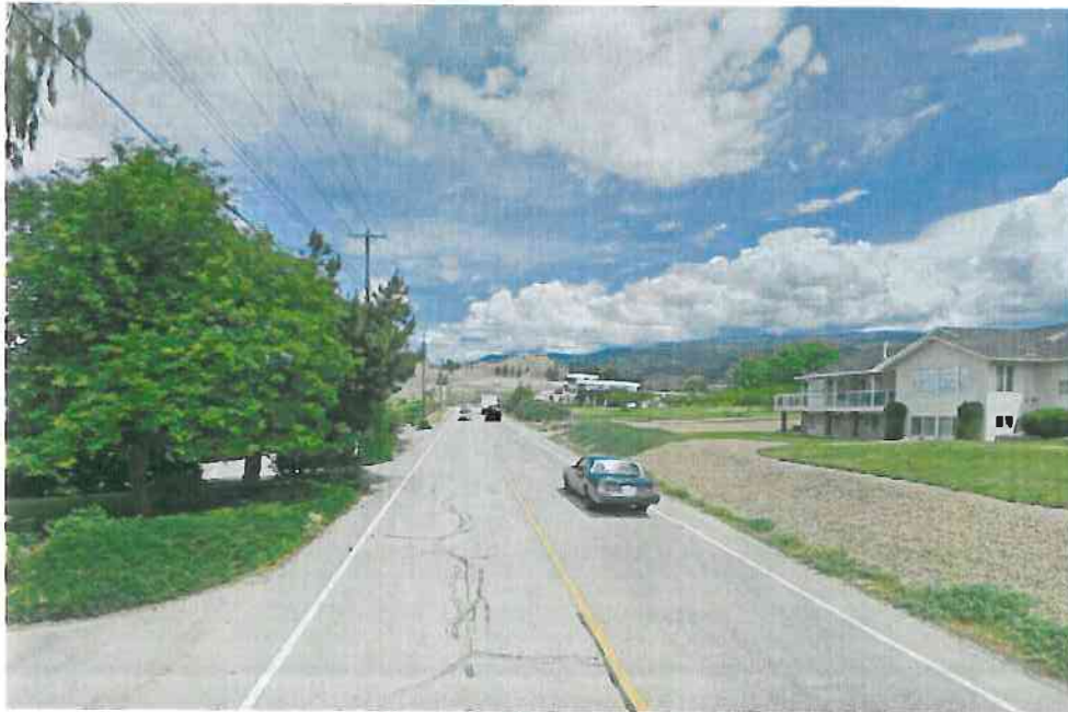
Figure 3: Existing Lower Bench Road (near Bankview Road)
