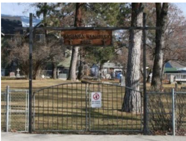
Figure 65: Repaint the main entry gate
