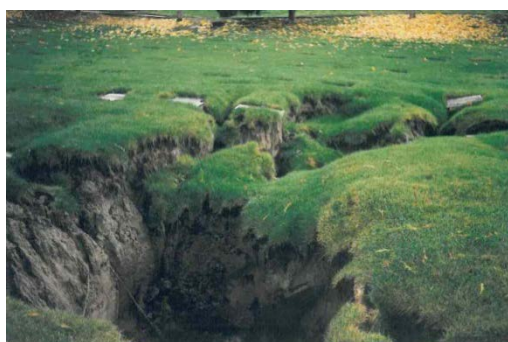
Figure 15: Effects of subsidence in 1997 (Source: City of Penticton)
