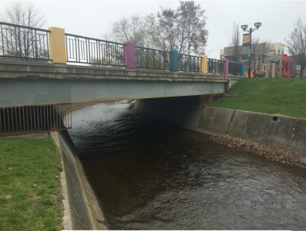
LOOKING UPSTREAM AT FRONT ST. BRIDGE
