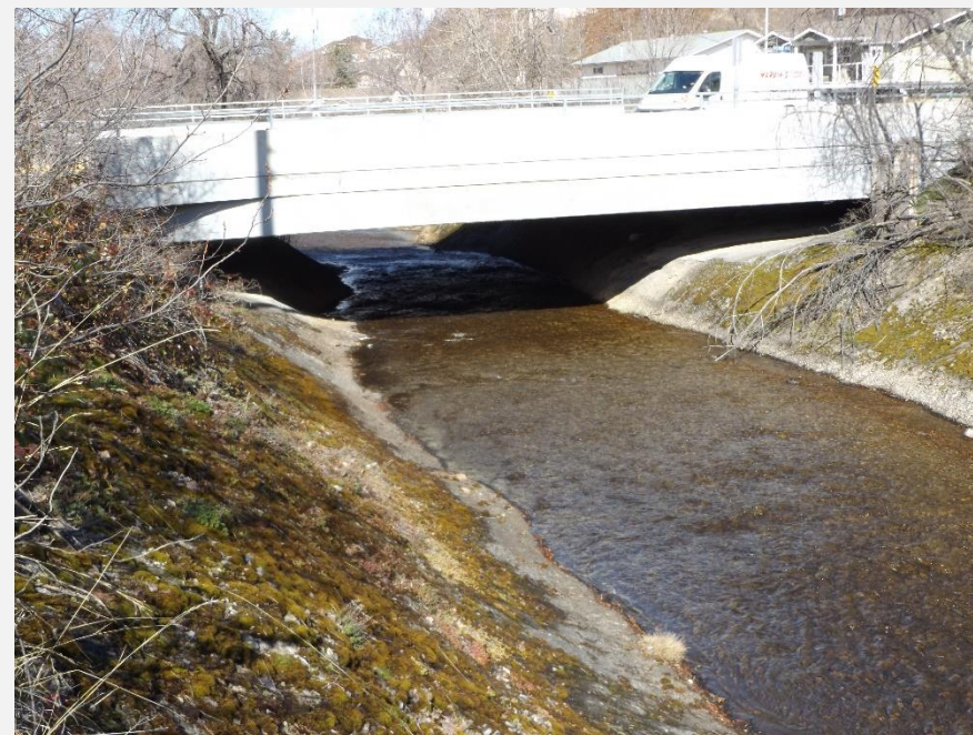
Looking downstream at Eckhardt Avenue bridge
