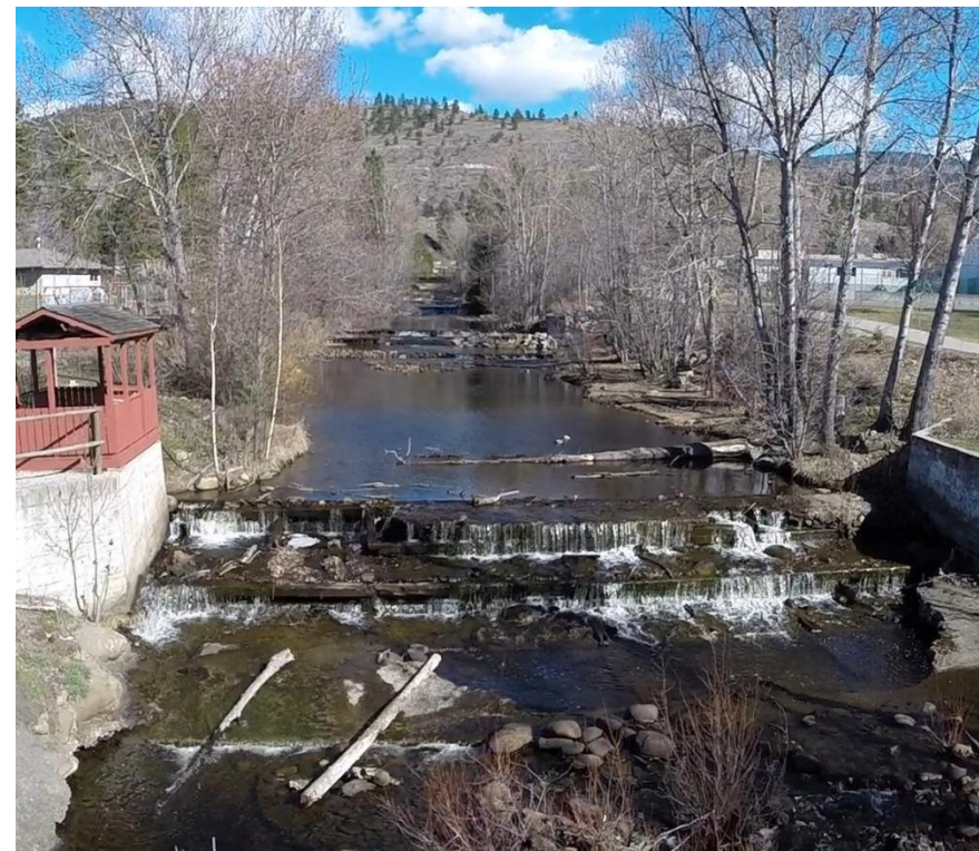
Section 2 – Stepped Channel
