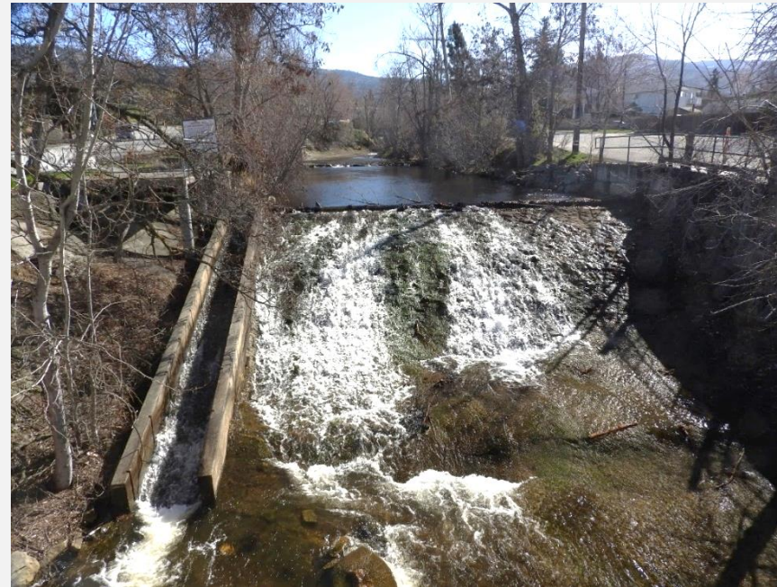
Looking upstream at Structure #2, From Wade Avenue Pedestrian Bridge
