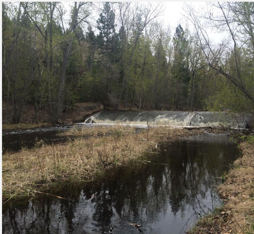
View of a structure, looking upstream
