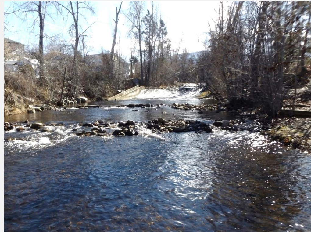
Looking upstream from Structure #2
