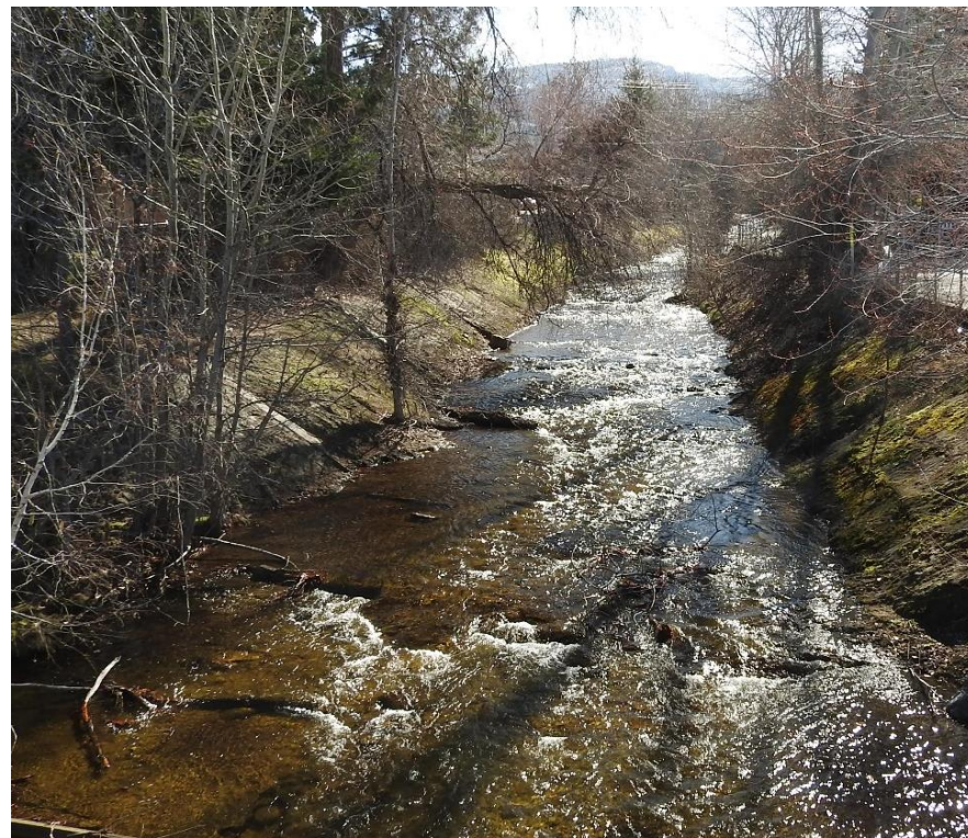
Section 1 – Concrete Lined
