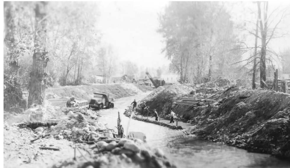
Construction of concrete lining. (Source Unknown)
