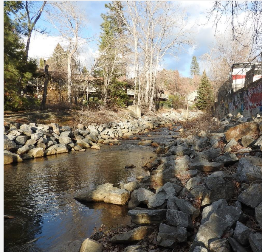
Looking upstream at Reach 9
