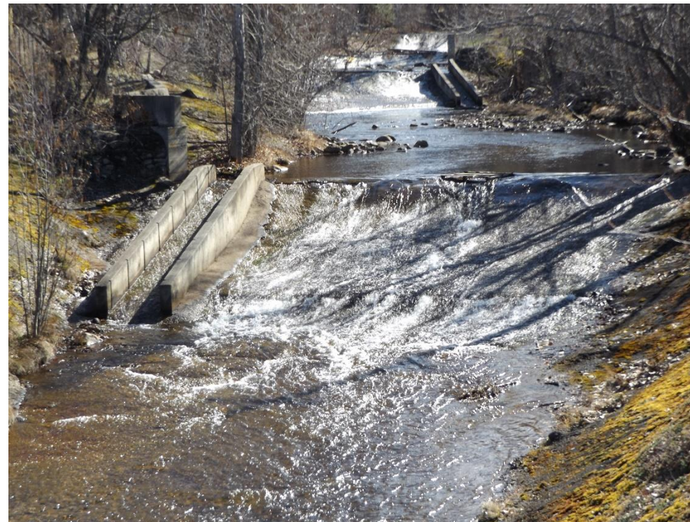
Drop Structure with Concrete Crest and Apron
