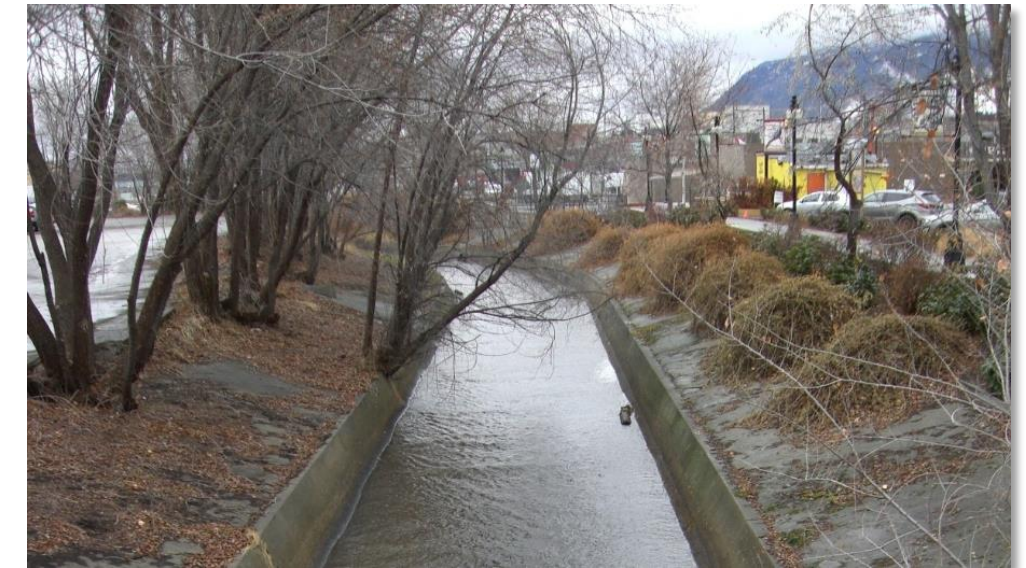
Penticton Creek below Ellis St. bridge (looking upstream)
