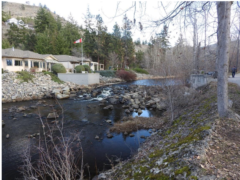
Drop Structure with Riprap Apron
