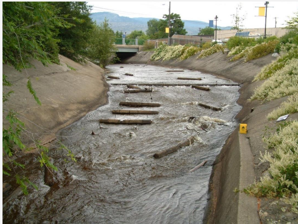
Looking upstream at Structure #1
