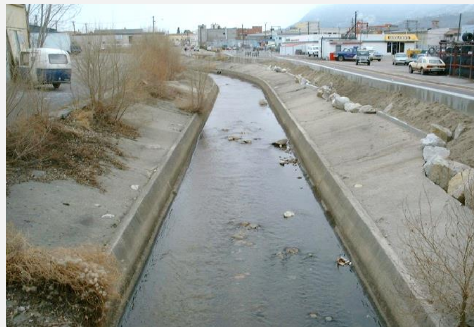
Formed concrete lining, facing upstream
