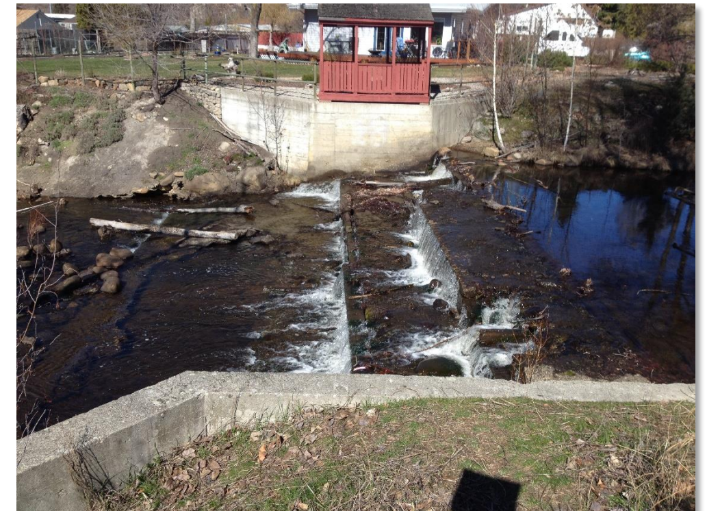
Wood Crib Drop Structure with Rock and Concrete
