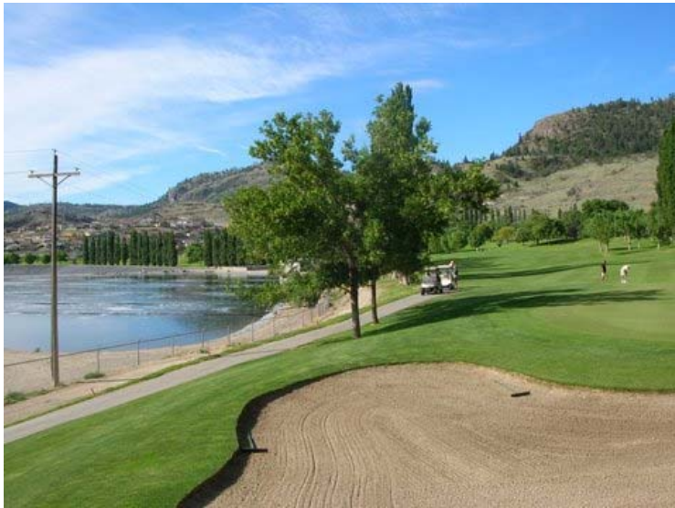
Osoyoos Golf Course and Treatment Plant
