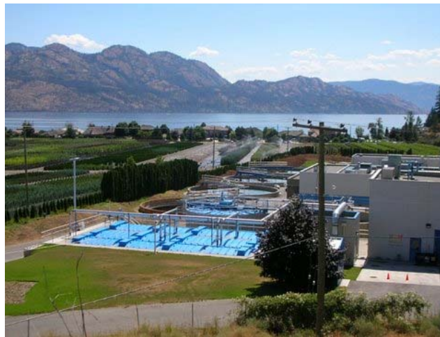
Westside Regional Wastewater Treatment Plant
