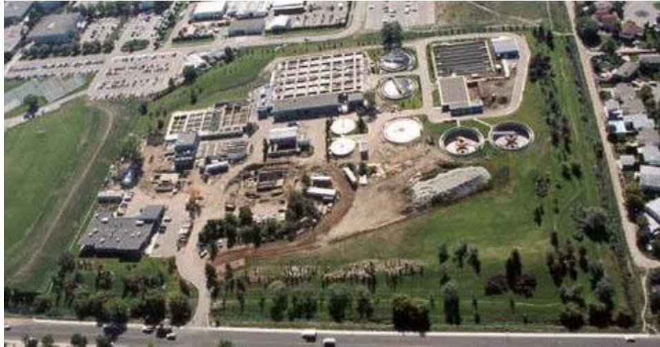
City of Kelowna Wastewater Treatment Plant
