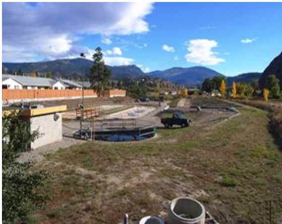
Okanagan Falls Sewage Treatment Plant
