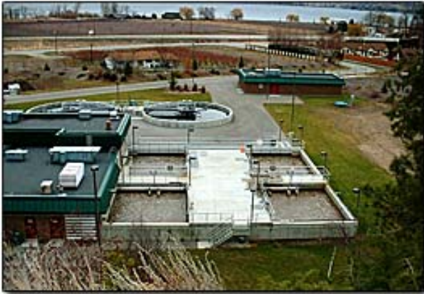
Summerland Wastewater Treatment Facility
