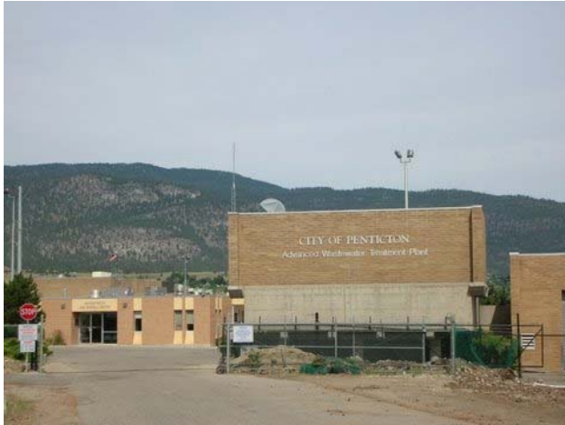
Penticton Wastewater Treatment Plant
