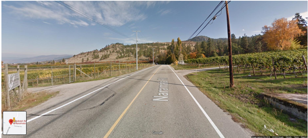
FIGURE 10 NARAMATA ROAD 100 M NORTH OF RANDOLPH ROAD (GOOGLE STREET VIEW)
