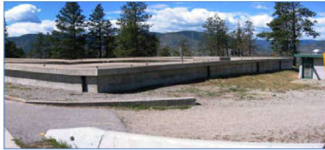
Duncan Avenue Reservoir
