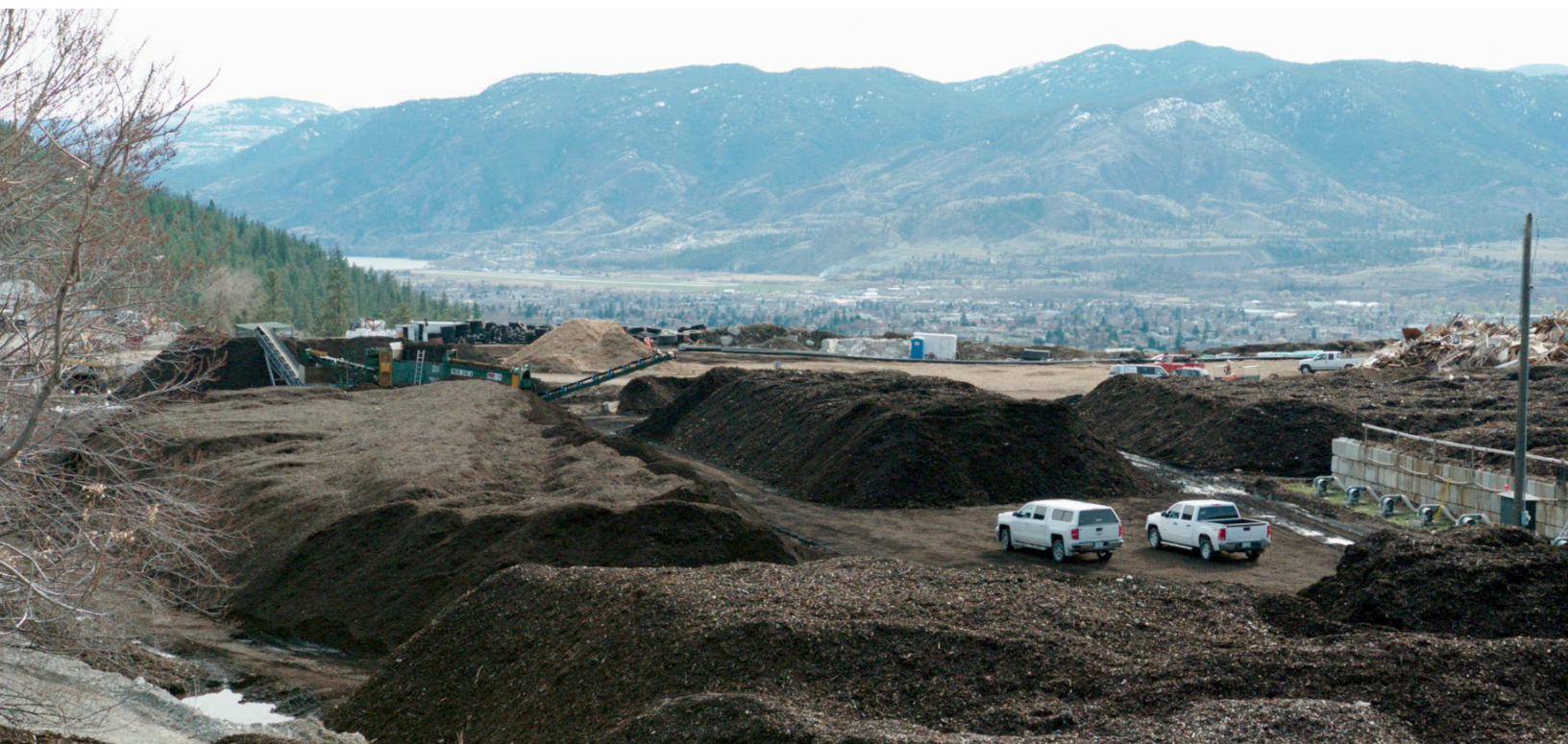
The solids from Penticton's waste water treatment process are composted at the Campbell Mountain Landfill.
