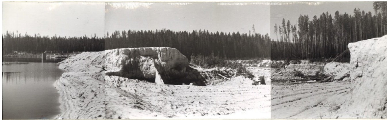
Breach of Ellis Creek No. 4 Dam (May 1941)
