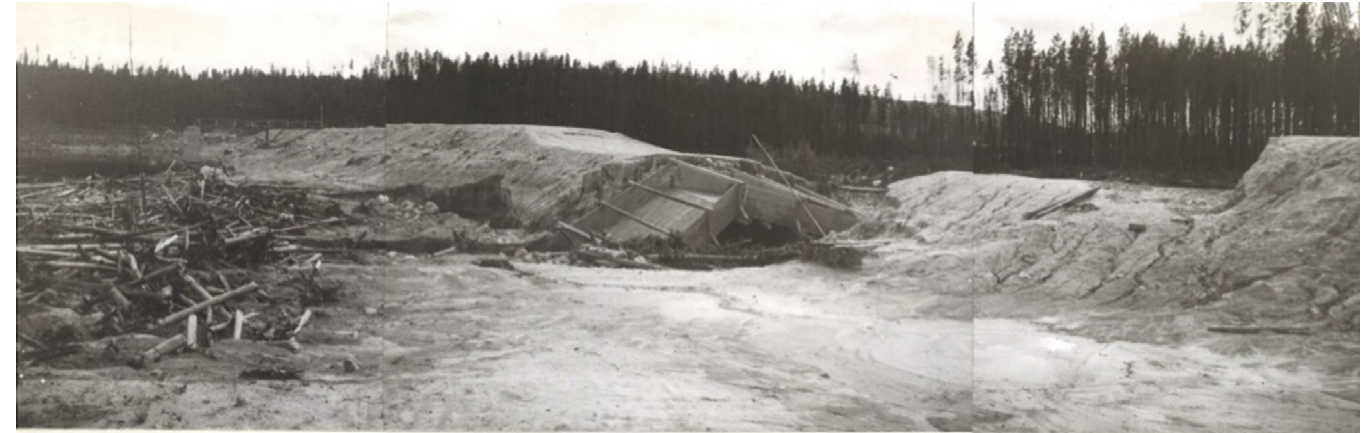
Breach of the Temporary Timber Spillway on Ellis Creek No. 4 Dam (May 1942)
