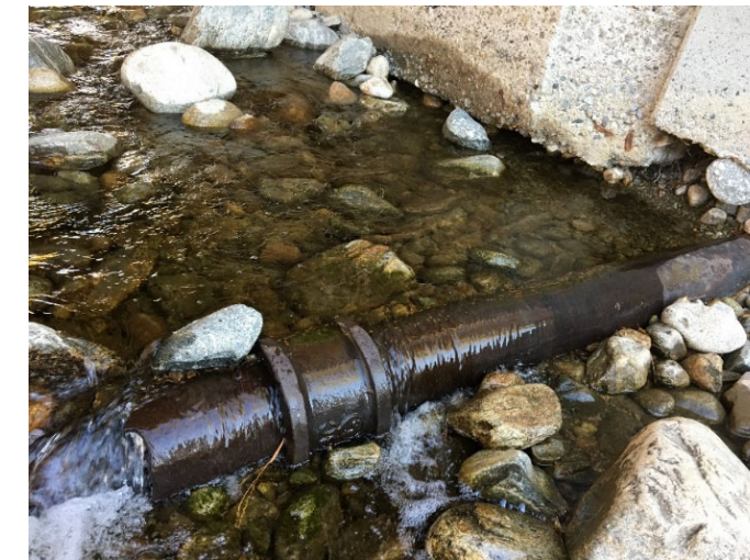
Exposed Pipe Upstream from Dartmouth Road Bridge
