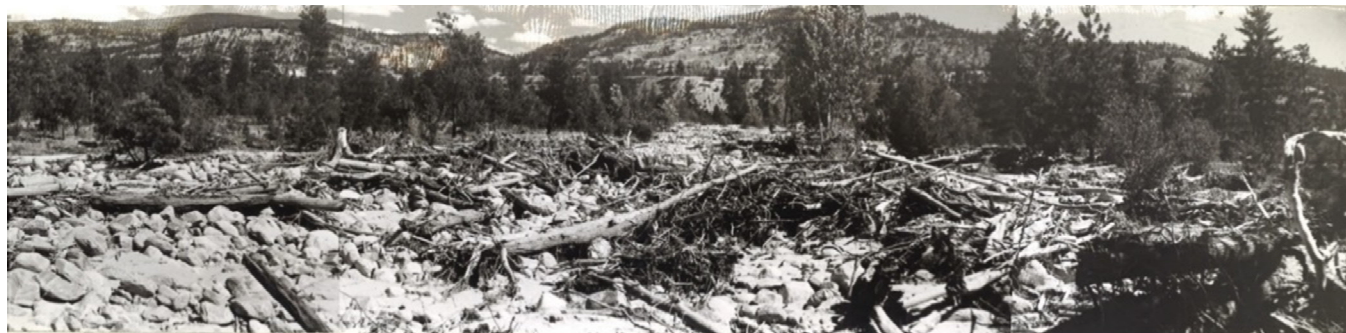
Flood Damage on IR2 From the Breach of Ellis Creek No. 4 Dam (May 1941)
