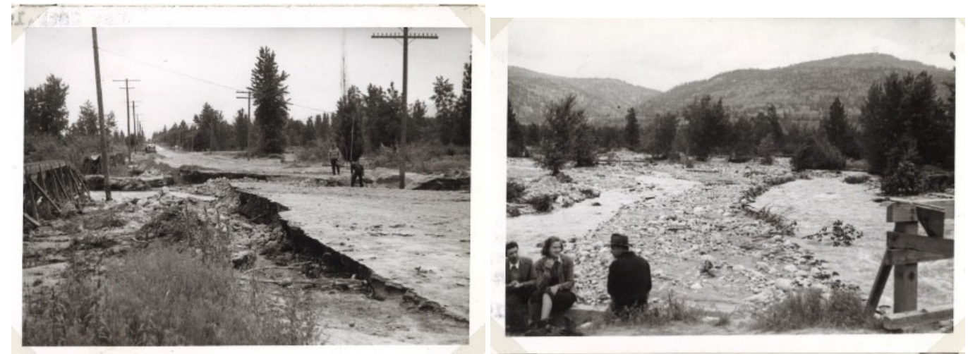
Resulting Flood Damage Downstream of Breach on Ellis Creek No. 4 Dam (May 1942)
