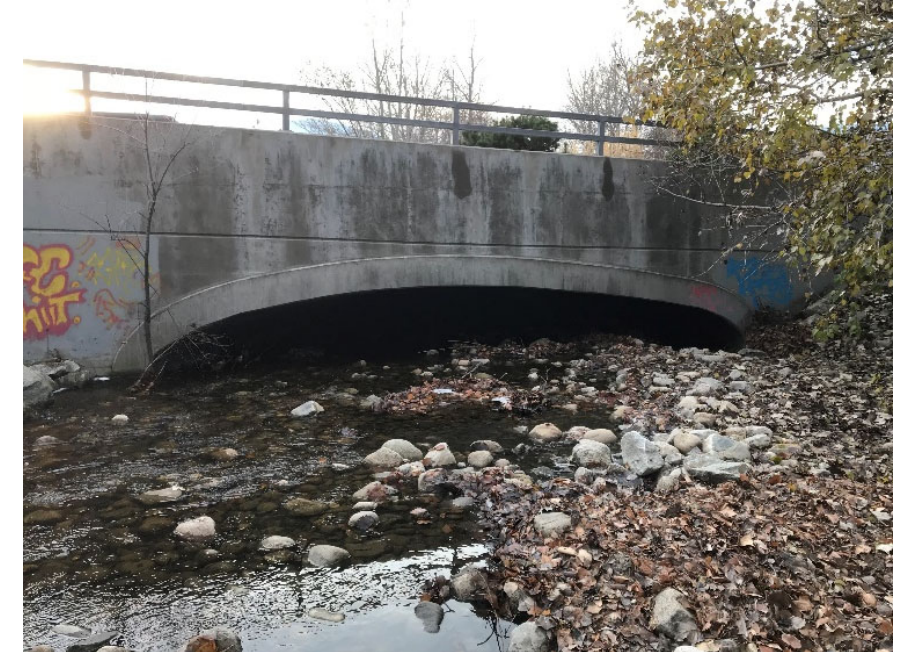
Aggradation in Ellis Creek Channel (Industrial Avenue Bridge)
