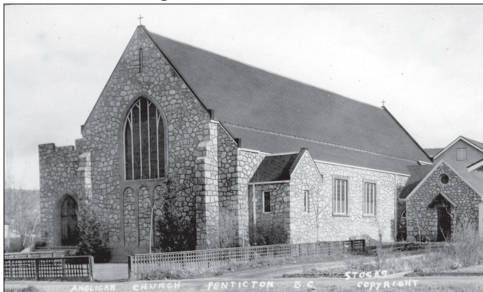
St. Saviour's Anglican Church on Orchard Ave. and Winnipeg St., 1930 PMA4443
