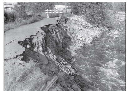
Ellis Creek flood damage in 1981 PMA8231
