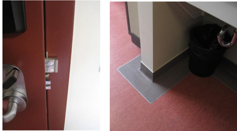
Figure 2: Examples of durable flooring & door hardware, Rock Bay Landing
