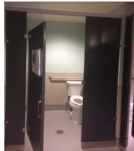
Figure 3: Example of accessible washroom, 3030 Gordon
