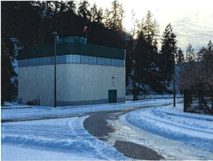
Figure 9: Residual Handling Building
