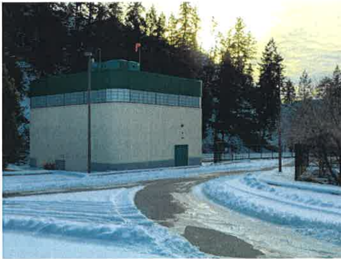
Figure 9: Residual Handling Building
