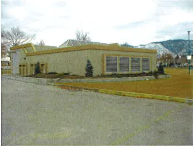
Figure 4: Penticton Creek Dam 2
