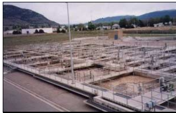
Advanced Waste Water Treatment Plant
