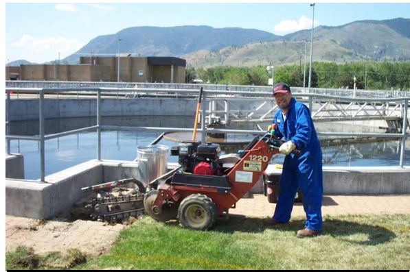
Work on the Waste Water Plant Treatment
