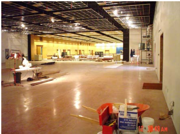
Convention Centre Renovations
