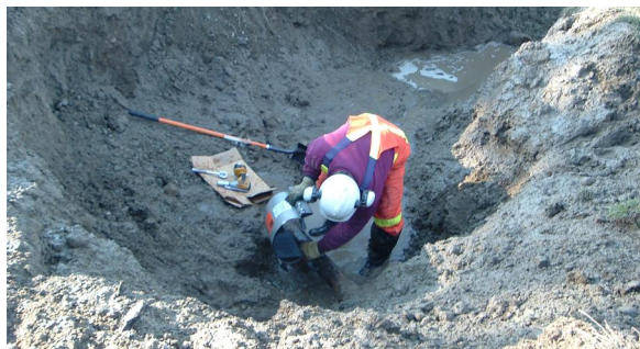
Repairing a Water Break
