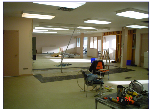
SECOND FLOOR RENOVATIONS
