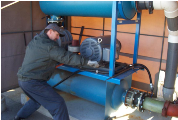
Repairs at the Waste Water Plant
