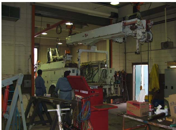
Digger Derrick Boom Repair
