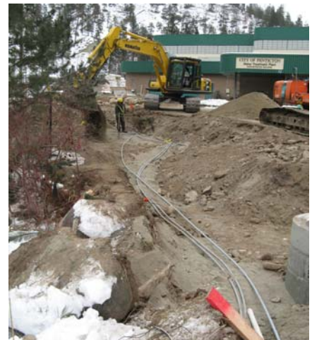
Water Treatment Plant Upgrade
