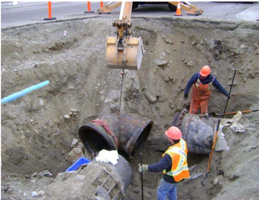
Forestbrook and Kilwinning 30" Pipe New Wash Bay
