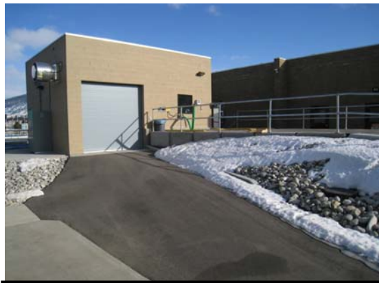
Septage Receiving Facility
