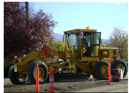
Road Grading Prior to Paving
