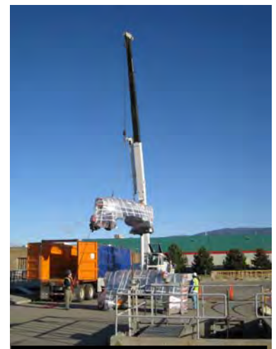
Unloading of new Centrifuges
