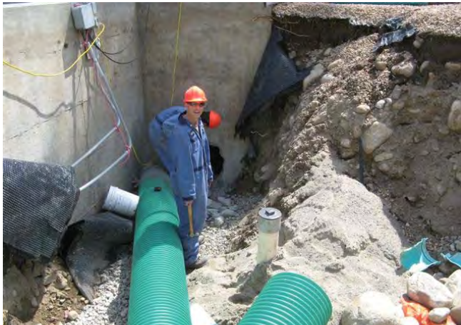
Installing filter to waste pipeline
