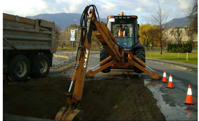
Fire Hydrant Installation
