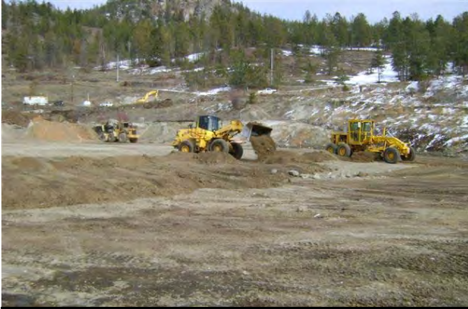
Grading Compost Site
