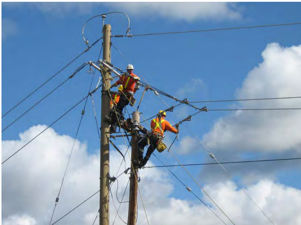
Power Line Technicians Tying in Conductors and Hardware
