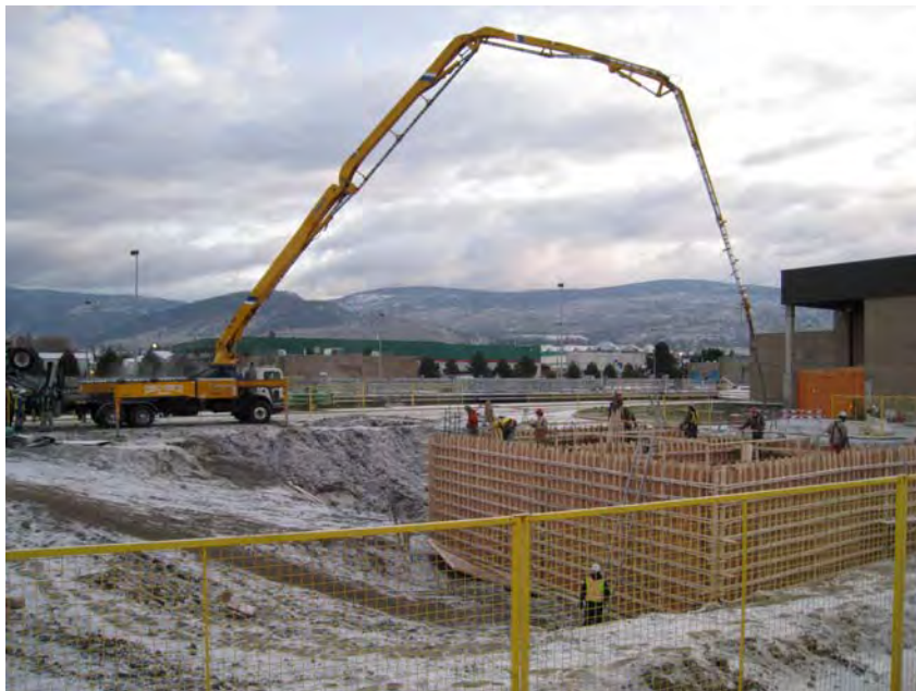
Pouring of Concrete for new dewatering building
