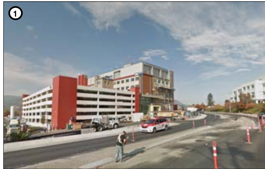
View of Government St. facing Penticton Regional Hospital
