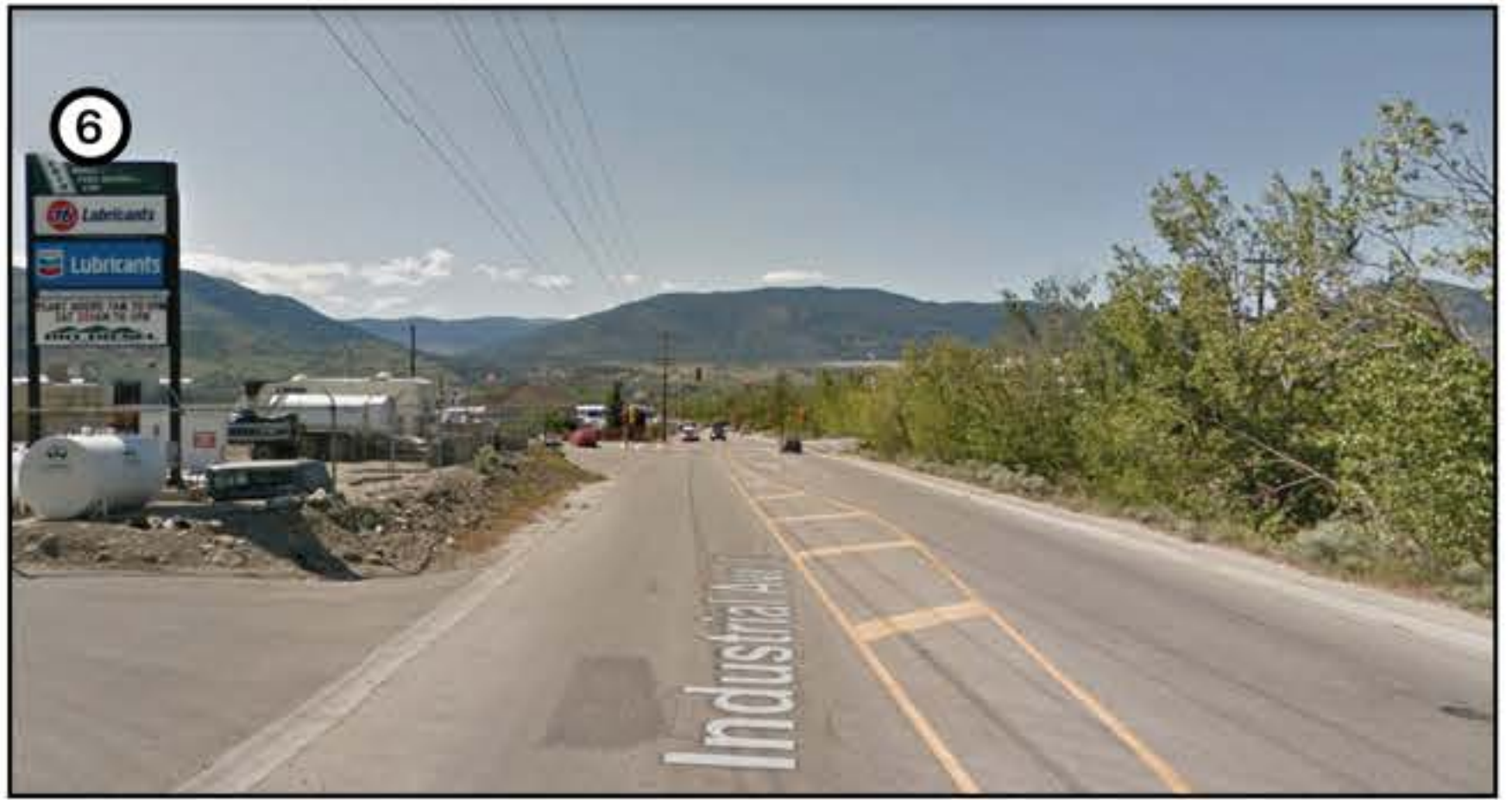
View of the south edge of the subject site, Industrial Ave facing west
