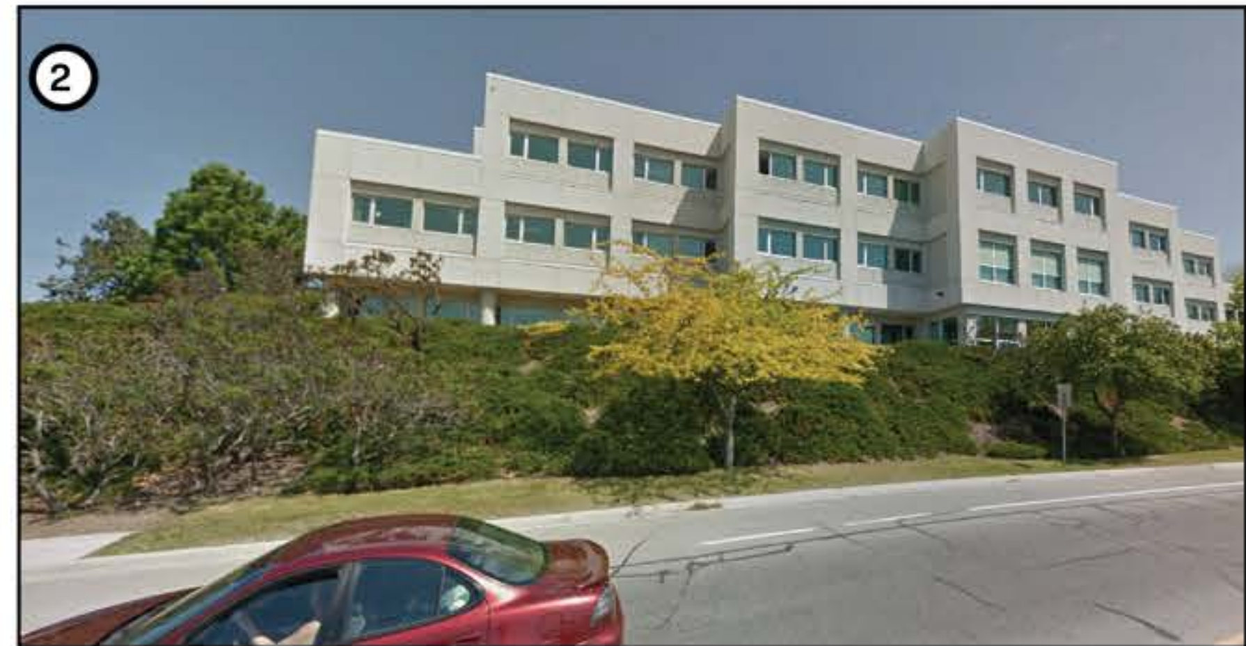
View of the 740 Carmi Ave, fronting onto Government St.
