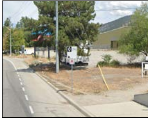
Figure 4 - New sidewalk will be installed along the Government St frontage to complete a sidewalk gap.
