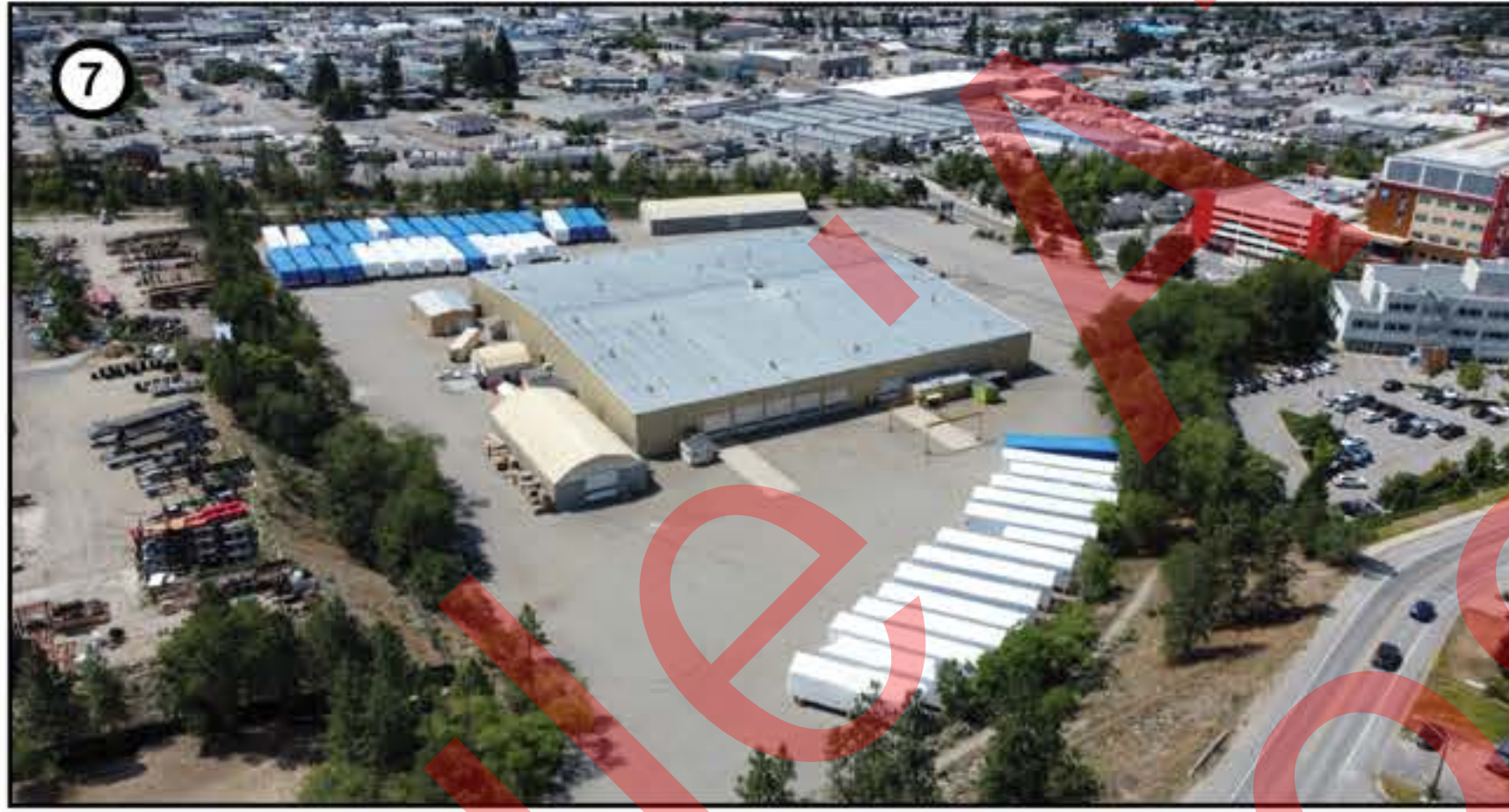
Drone shot of overall project site facing southwest
