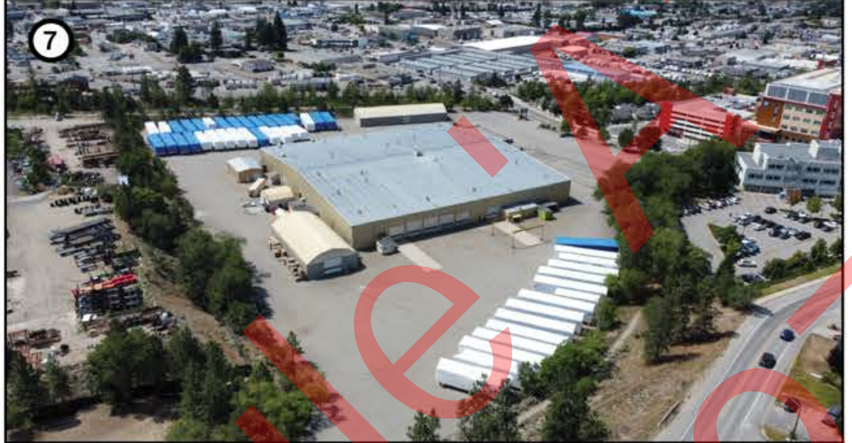
Drone shot of overall project site facing southwest
