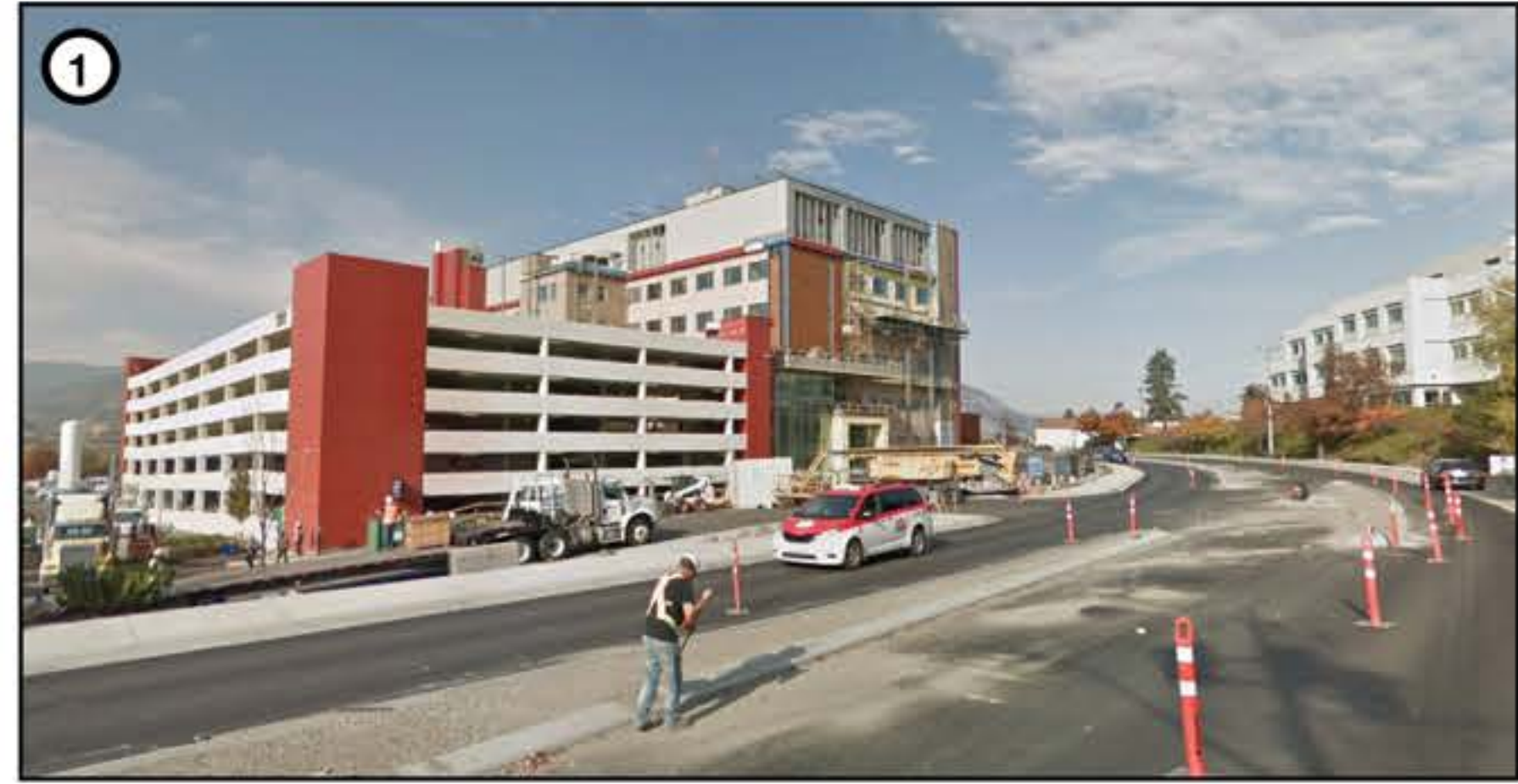
View of Government St. facing Penticton Regional Hospital
