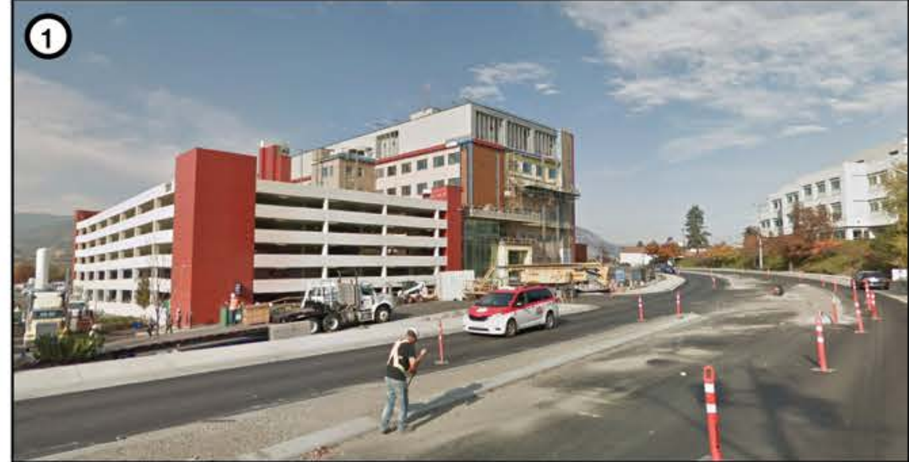
View of Government St. facing Penticton Regional Hospital
